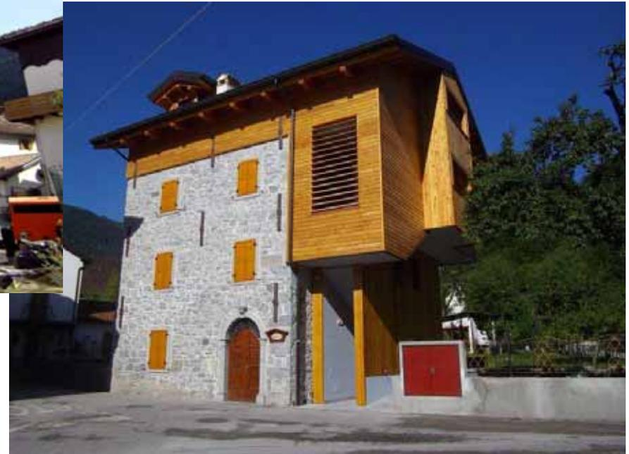
Tecnologie costruttive innovative – Sistema CLT – Cross Laminated Timber
