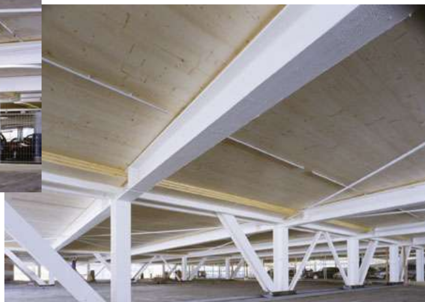
Garage multi piano – Innsbruck (Austria)
