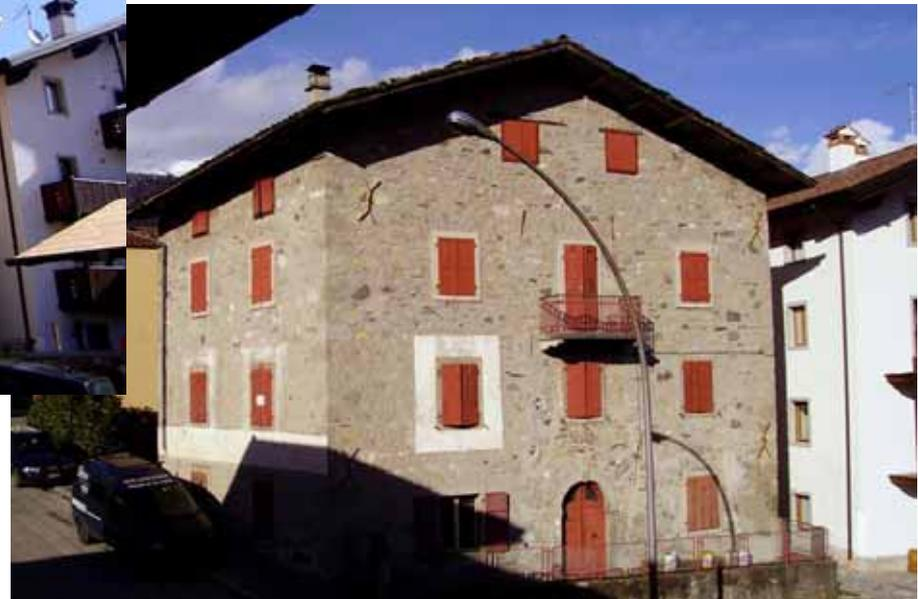
Comune di Sutrio (UD) 3487 GG –  $S_{Netta}=370\text{ mq}$  –  $S/V=0,60$  –  $PT_{Risc}=9,1\text{KW}$  –  $IE=34\text{ kWh/m}^2\text{a}$
