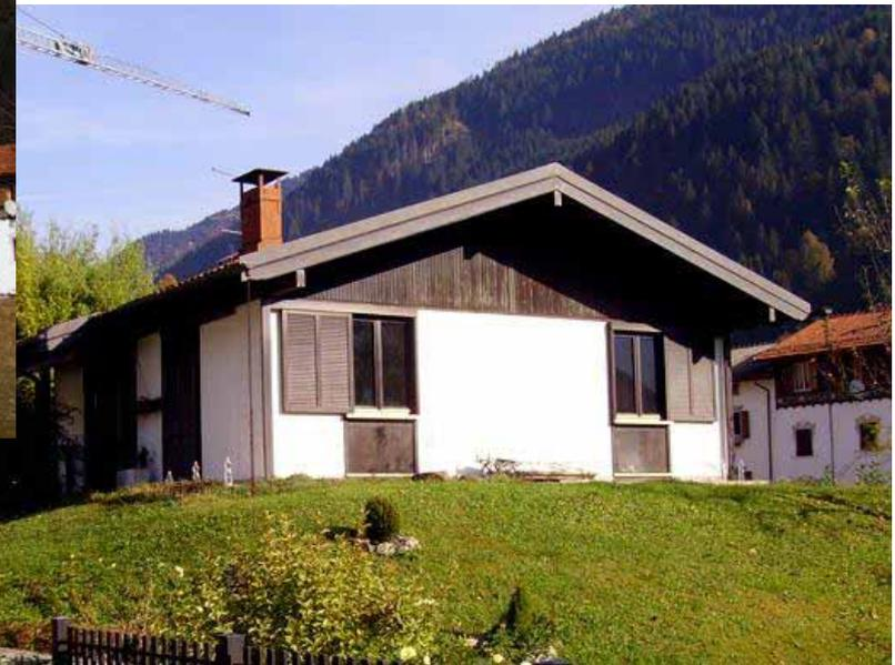
Comune di Paluzza (UD) 3297 GG –  $S_{Netta}=78$  mq –  $S/V=0,89$  –  $PT_{Risc}=4,8KW$  –  $IE=64$  kWh/m<sup>2</sup>a
