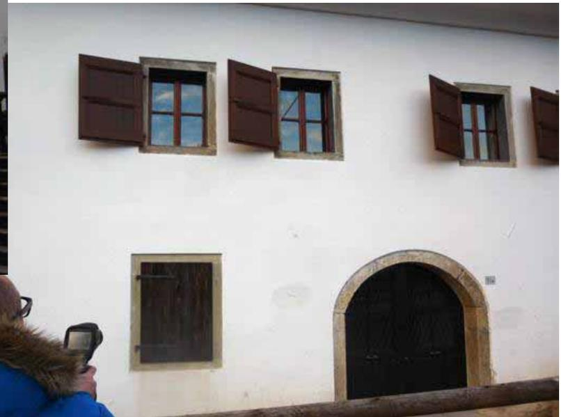
Comune di Ovaro (UD) 3386 GG –  $S_{Netta}=155\text{ mq}$  –  $S/V=0,66$  –  $PT_{Risc}=7,8\text{KW}$  –  $IE=68\text{ kWh/m}^2\text{a}$
