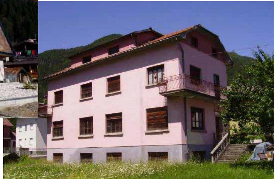
Comune di Paluzza (UD) 3297 GG –  $S_{Netta}=282\text{ mq}$  –  $S/V=0,63$  –  $PT_{Risc}=8,7\text{KW}$  –  $IE=21\text{ kWh/m}^2\text{a}$
