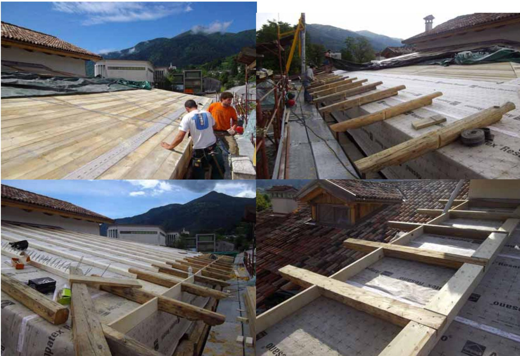
SCHEMA DI POSA DELLA COPERTURA CON TENUTA ALL'ARIA INTERNA E TENUTA AL VENTO ESTERNA
