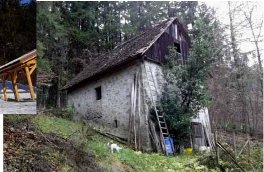
Comune di Sutrio (UD) 3487 GG –  $S_{Netta}=80\text{ mq}$  –  $S/V=0,87$  –  $PT_{Risc}=2,5\text{KW}$  –  $IE=45\text{ kWh/m}^2\text{a}$
