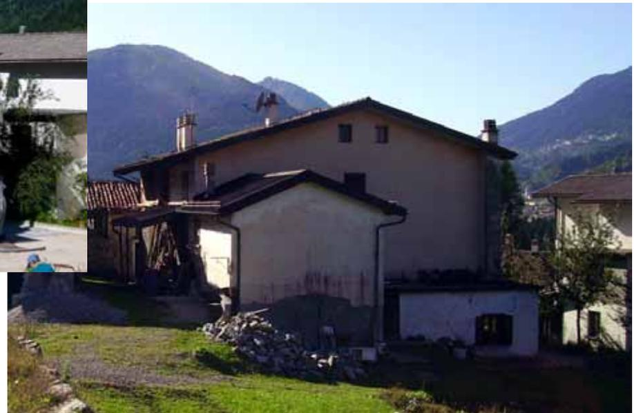
Comune di Paluzza (UD) 3297 GG –  $S_{Netta}=336$  mq –  $S/V=0,73$  –  $PT_{Risc}=12,5$  KW –  $IE=40$  kWh/m<sup>2</sup>a
