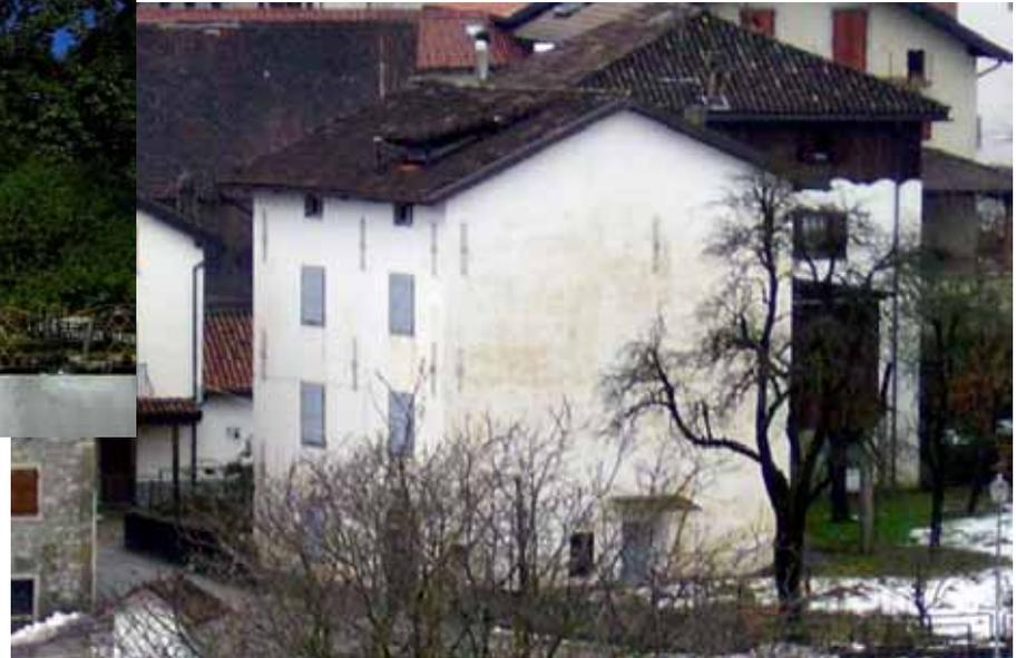
Comune di Sutrio (UD) 3487 GG –  $S_{Netta}=334\text{ mq}$  –  $S/V=0,62$  –  $PT_{Risc}=8,2\text{KW}$  –  $IE=49\text{ kWh/m}^2\text{a}$
