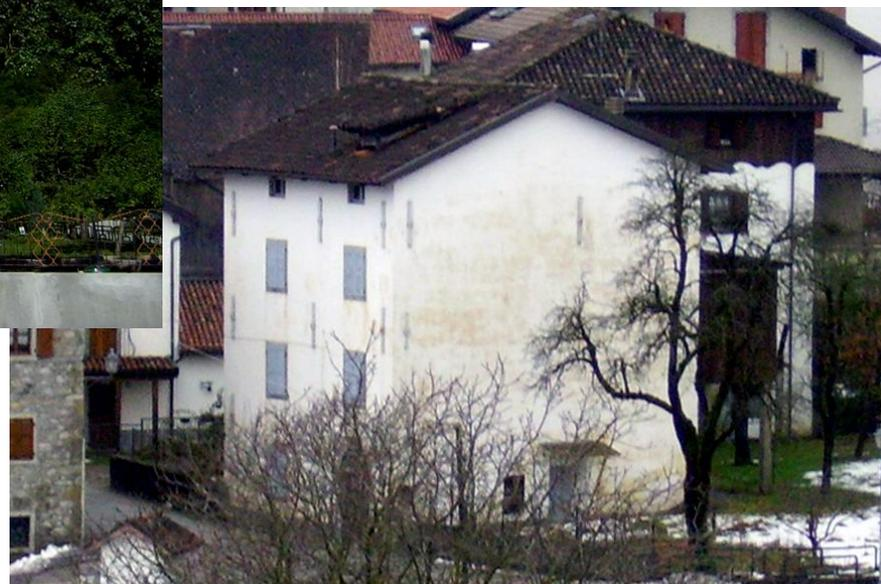
Comune di Sutrio 3487 GG –  $S_N=334 \text{ mq}$  –  $S/V=0,62$  –  $PT_R=8,2 \text{ KW}$  –  $IE=49 \text{ kWh/m}^2\text{a}$  = 4,9 LtGas/McMet/m<sup>2</sup>a
